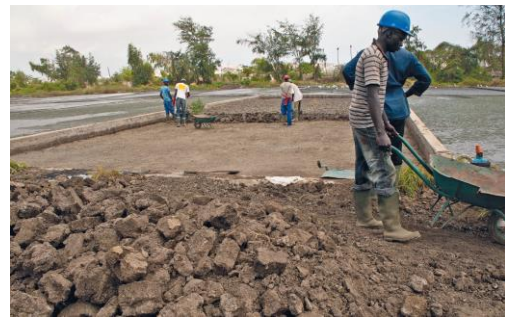
Fig. 1. Extracting sludge from the unplanted drying beds at the Cambérène treatment facility in Dakar, Senegal (Dodane and Ronteltap, 2014)
