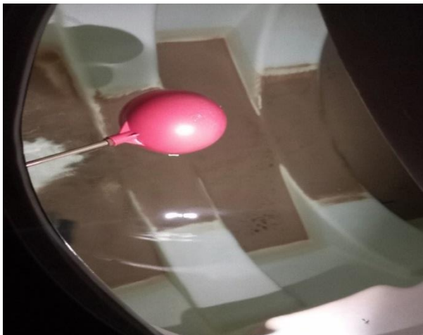
Fig. 9. An example of sediment accumulation at the bottom of the cistern
