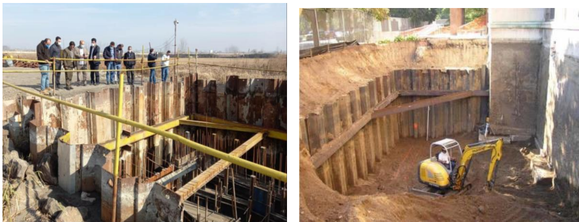
Fig. 3. Sheet pile Wall (Kara Azmoon Sazeh Azma, 2020)
