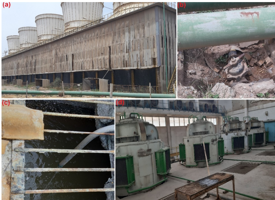
Fig. 1. a) Cooling tower, b) bleach injection line, c) H_2SO_4 injection line and d) pumps for transferring water to condenser
