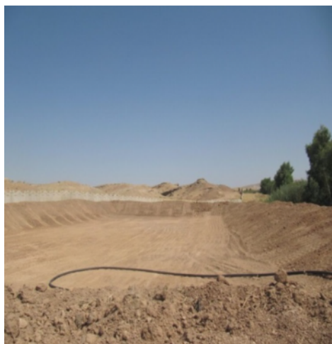
Fig. 2. Construction of an earthen pool at the treatment plant
