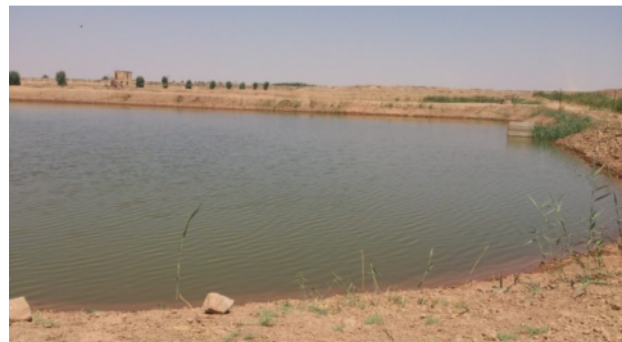
Fig. 4. Pool dewatered by wastewater treated by Wetland method
